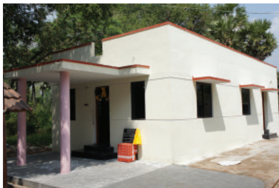
The New Dining Area
